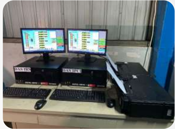
Isntalasi System DAS (PLTU Indorama Polychem)
